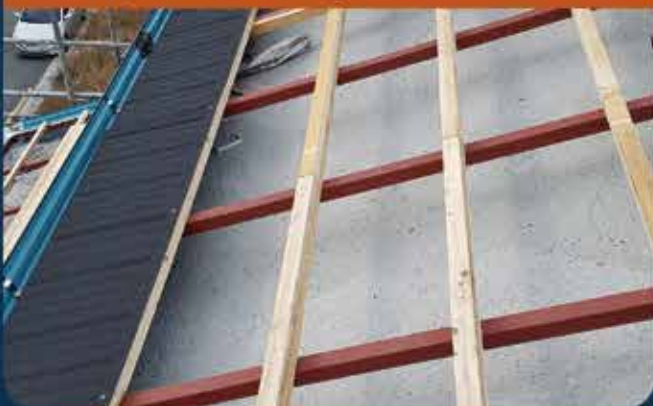
🕒 Installation of gutter and eaves
