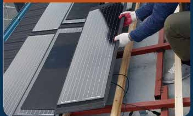
🕒 Installation of JASCO Solar Roof Tiles
