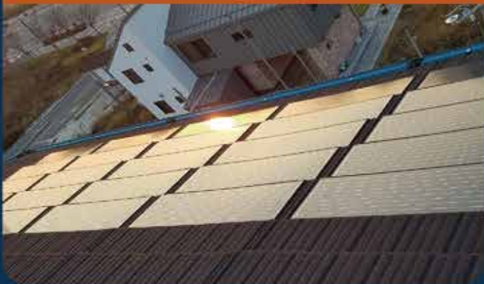
④ Installation and finishing of edges of solar roof tiles
