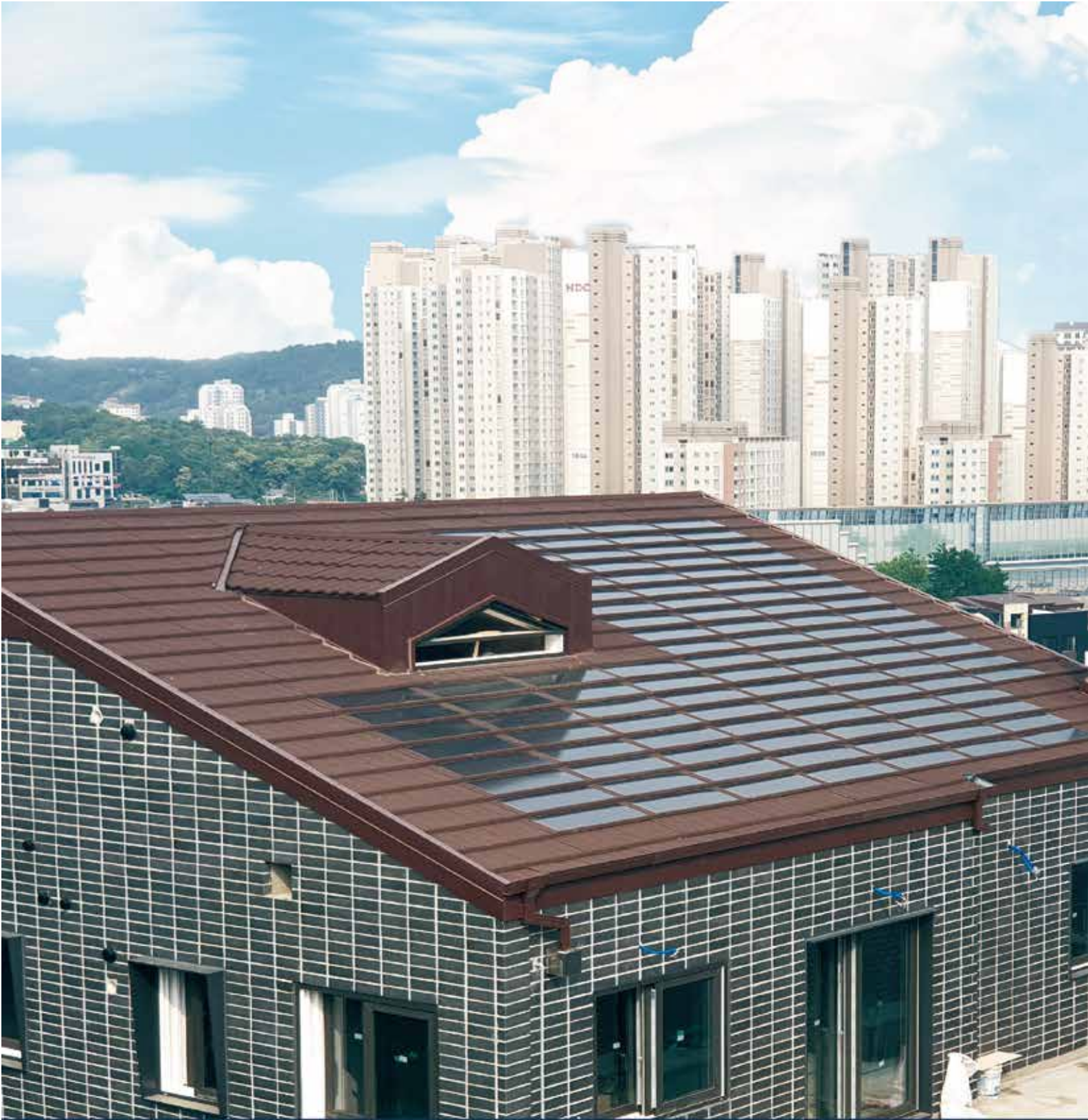
④ Installation and finishing of edges of solar roof tiles
